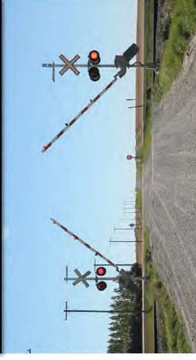
Example: Signalized Grade Crossing
