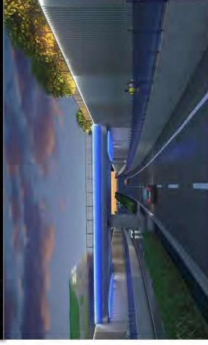
Example: Urban Road/Rail Grade Separation
